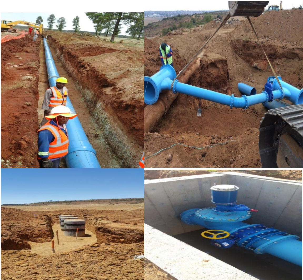
Vista Park 2 & 3 : Realignment of bulk water and sewer line
