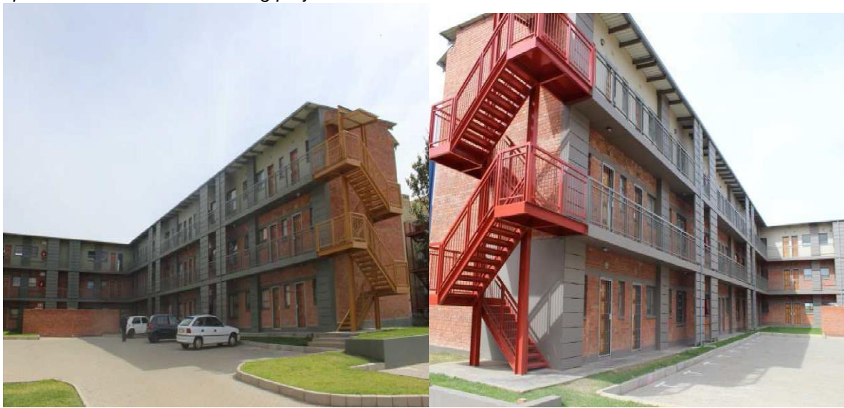
Completed Units of the Brandwag Social Housing Project
